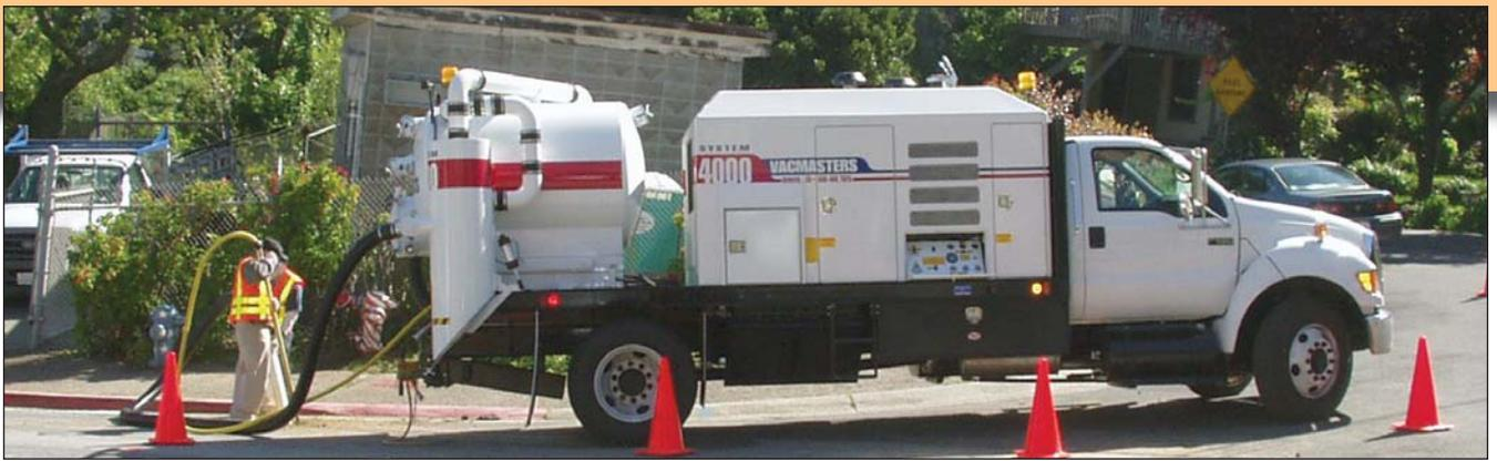
iameter, 8-foot-deep pile holes for a concrete foundation located in close proximity to buried gas and electric utilities.
